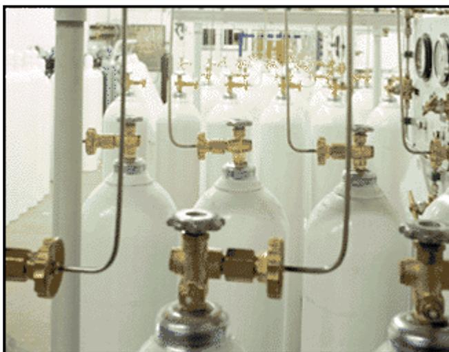
The labels should be color coded to distinguish hazardous gases (such as flammable, toxic, or corrosive substances) (e.g., a yellow background and black letters).
